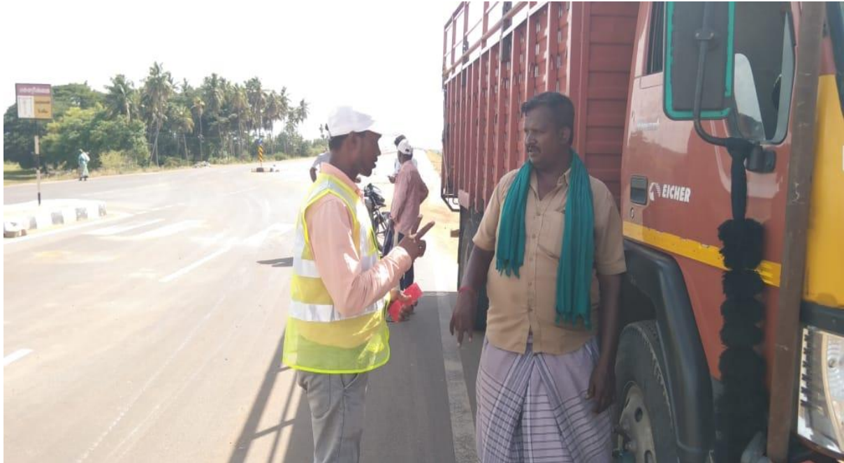
Safety instructions given to Drivers and Reflecting stickers pasting at Ch. 140+100
